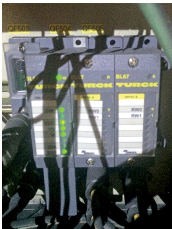
All data from the read/write heads converges at the BL67 gateway and the RFID-S modules
